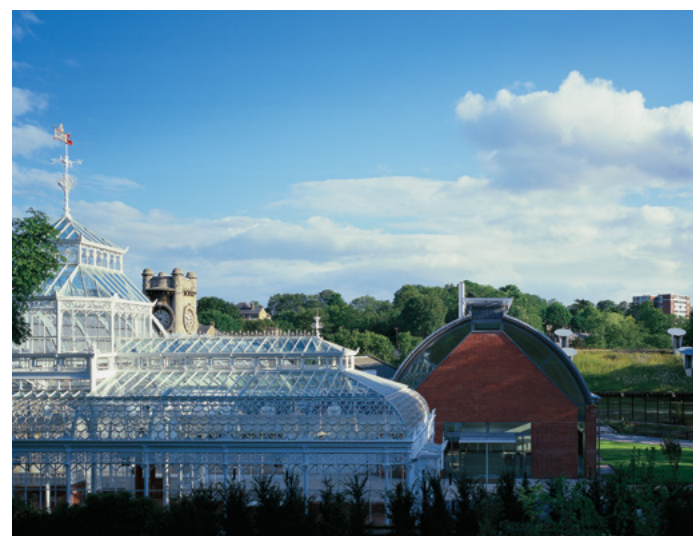
Horniman Museum conservatory, museum extension and timber Conservation Centre with green roof (Allies and Morrison / Peter Cook)
