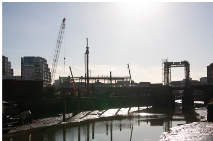
Construction site in Deptford
