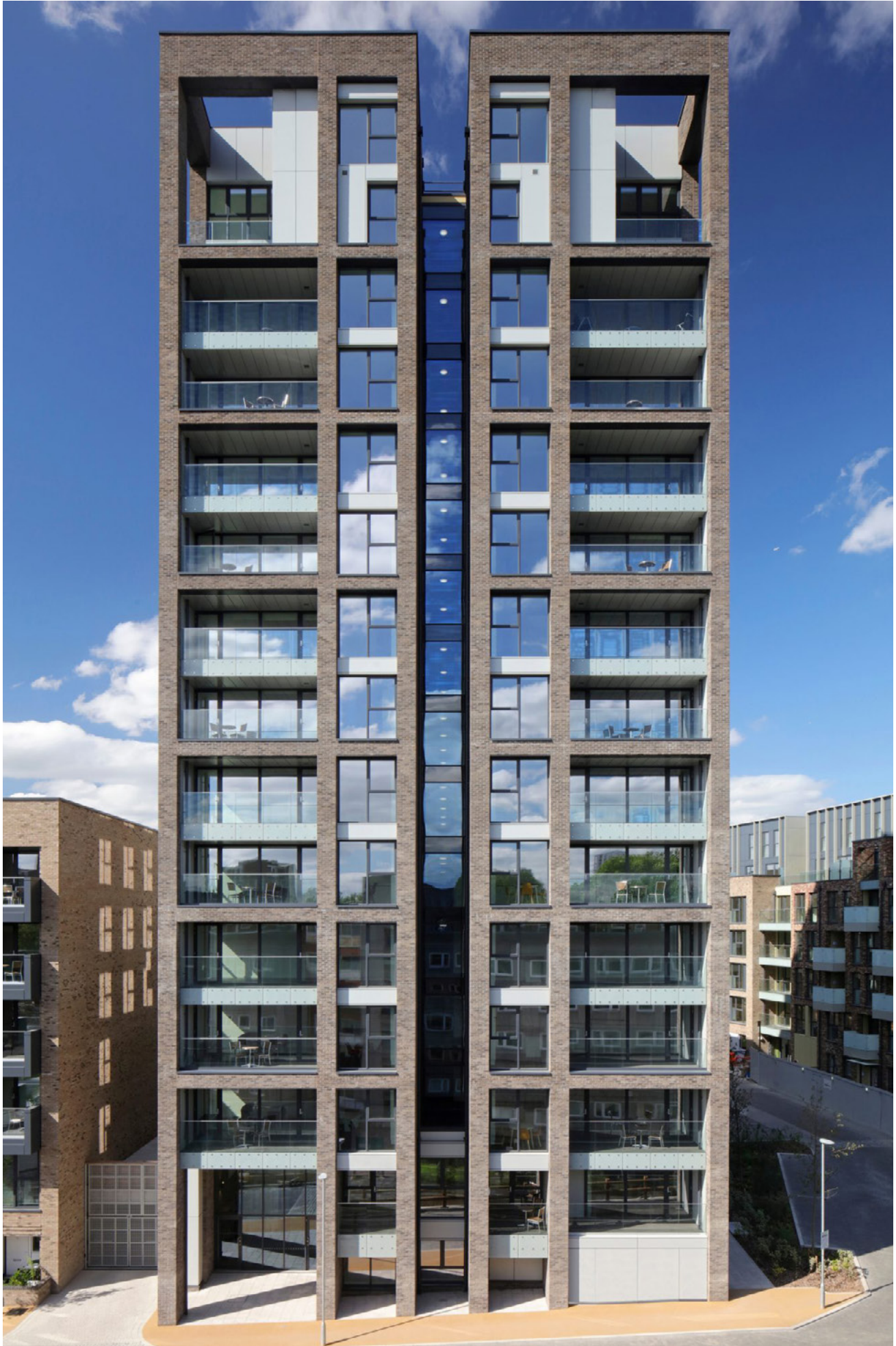
New development at Heathside and Lethbridge (BPTW)
